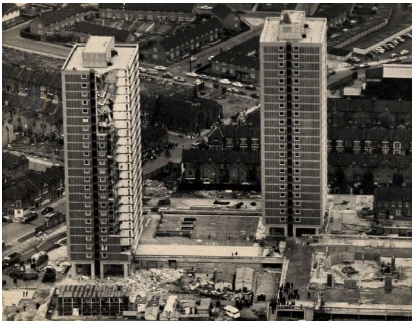
Figure 2-2: Partial collapse of Ronan Point Tower (left) London, 1968 (Daily Mail)
